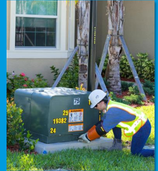
Putting more power lines underground
